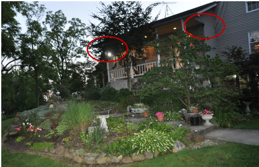
Figure 5: Front view of residence – Video Camera locations circled
